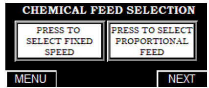
Figure 8. Chemical Feed Screen
